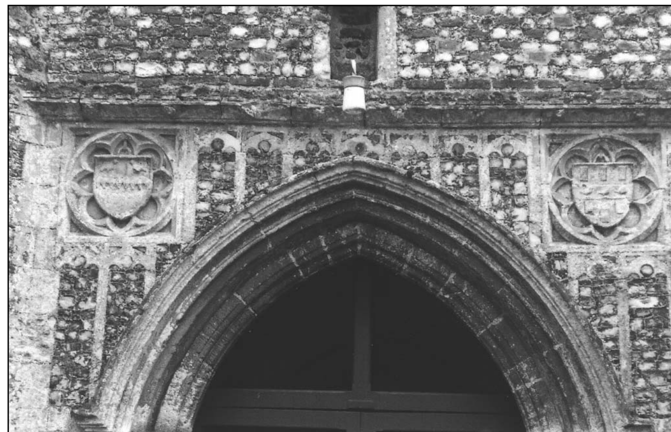
Figure 11. North porch of the church showing the Irmingland and Daubeney shields.
